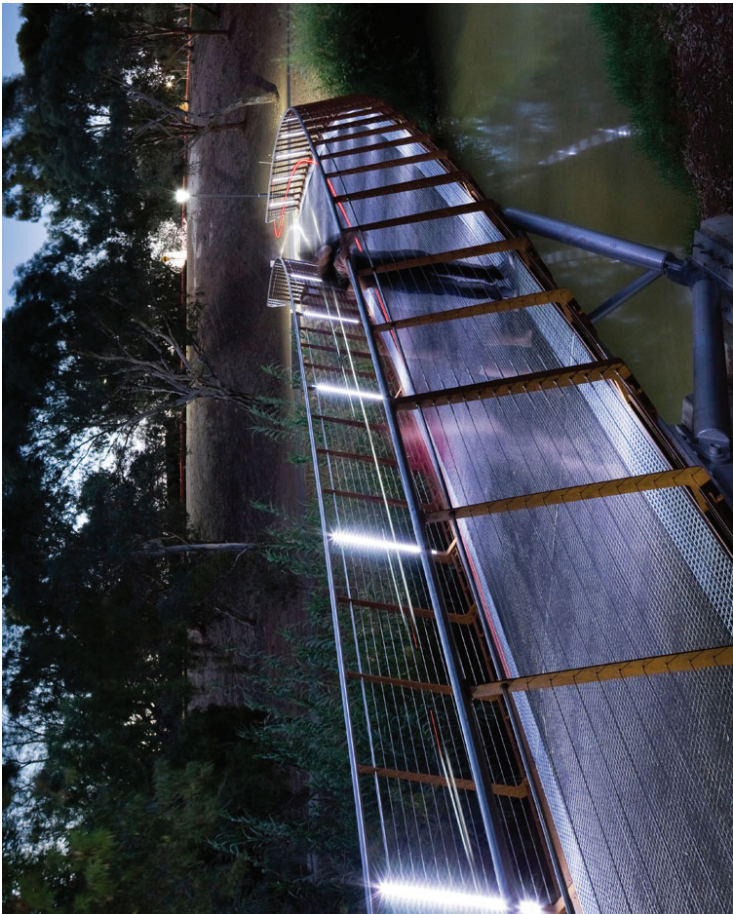
Integrated Rail Lighting at Bridges, Stairs and ADA Ramp
